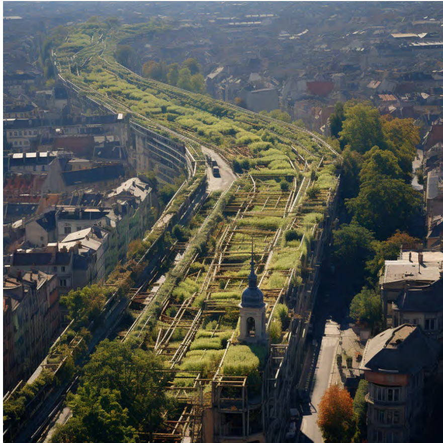
The Gürtel literally transformed into a green belt around the central districts.
